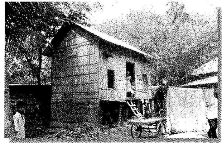
Figure 3: A CCDB mini-community flood-shelter
